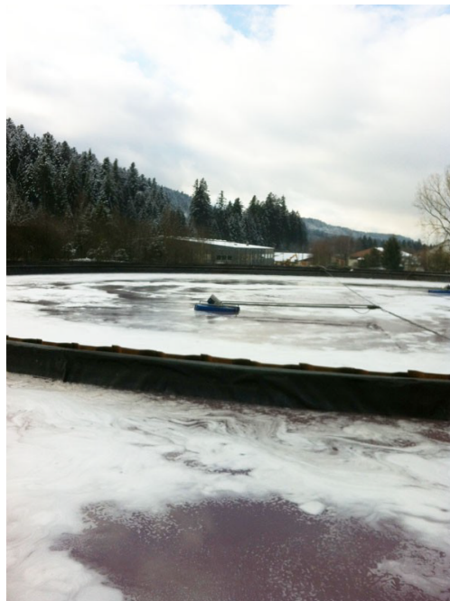
Buffer tank in a textile industry (5 HYDROPULSE 4kW)
